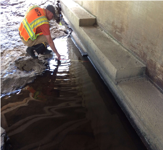
PHOTO 1 Description Bent 1 minor voids under edge of footing.
